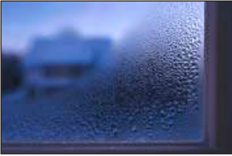
Condensation on the inside of a windowpane.
